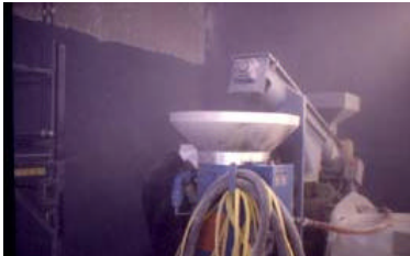
Figure 1. ARMS™ inside containment where wall decontamination is taking place.
