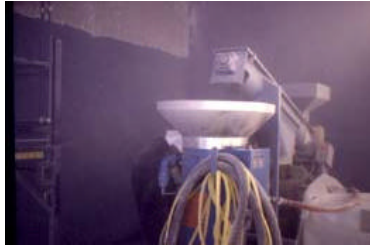
Figure 1. ARMS™ inside containment where wall decontamination is taking place.
