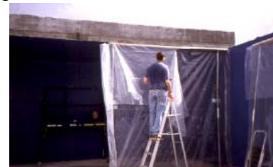
Figure 2. Containment being built around wall decontamination area.
