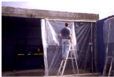
Figure 2. Containment being built around wall decontamination area.
