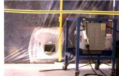
Figure 4. Filter unit in containment where wall decontamination is taking place.
