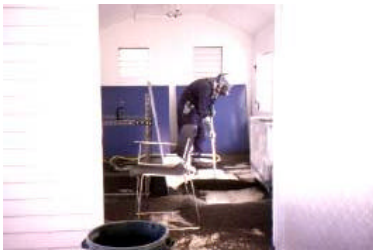
Figure 2. Worker inside shed blasting metal plate.
