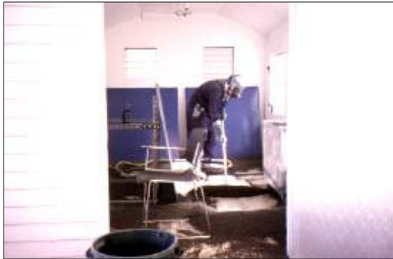
Figure 2. Worker inside shed blasting metal plate.
